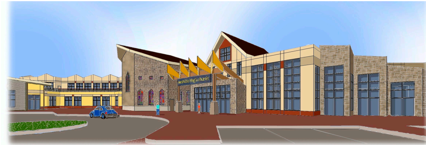
main entrance from south
